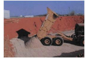
In 2003, over 3,700 tons of soils were excavated at the Adhesive Disposal Area to approximately 13 feet deep. Here a dump truck brings in material to continue backfilling. The backfill was placed in approximately 1-foot lifts and compacted.
